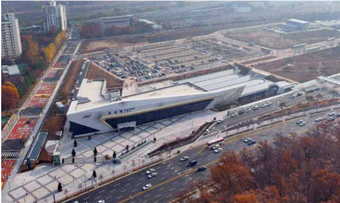
| Figure 4-3 | Suseo Station
