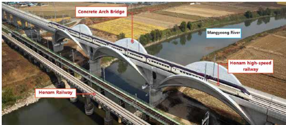
| Figure 2-8 | Panoramic view of the Mangyeong-gang River Bridge in Section 3-3 of the Honam high-speed railway
