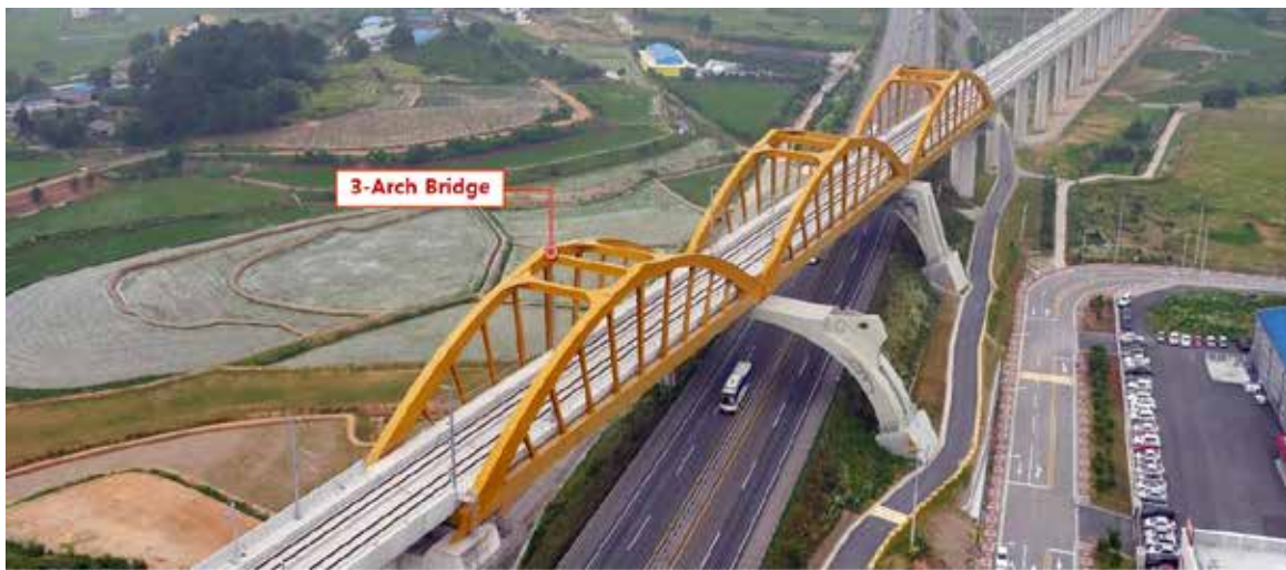
| Figure 2-7 | Panoramic view of Honam high-speed railway Section 2-3 overpass
