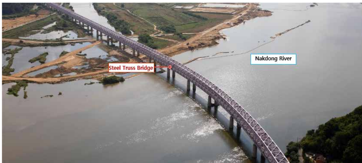
| Figure 2-3 | Panoramic view of the Nakdong River Bridge on the Gyeongjeon Line Samnangjin~Jinju double-track railway
