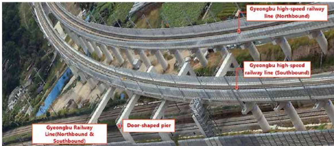
| Figure 2-9 | Panoramic view of the gate-shaped pier of Panam 1 Bridge in the Daejeon city center section of the Gyeongbu high-speed railway
