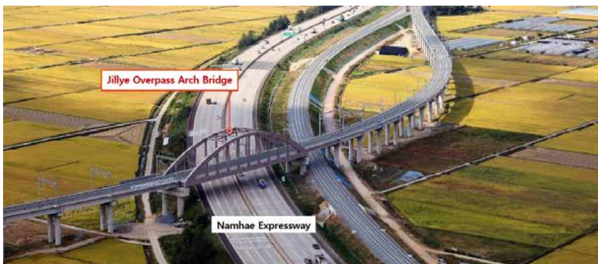
| Figure 2-4 | Panoramic view of Jinrye Overpass (Haroarch Bridge) on the Gyeongjeon Line Samnangjin~Jinju double-track railway
