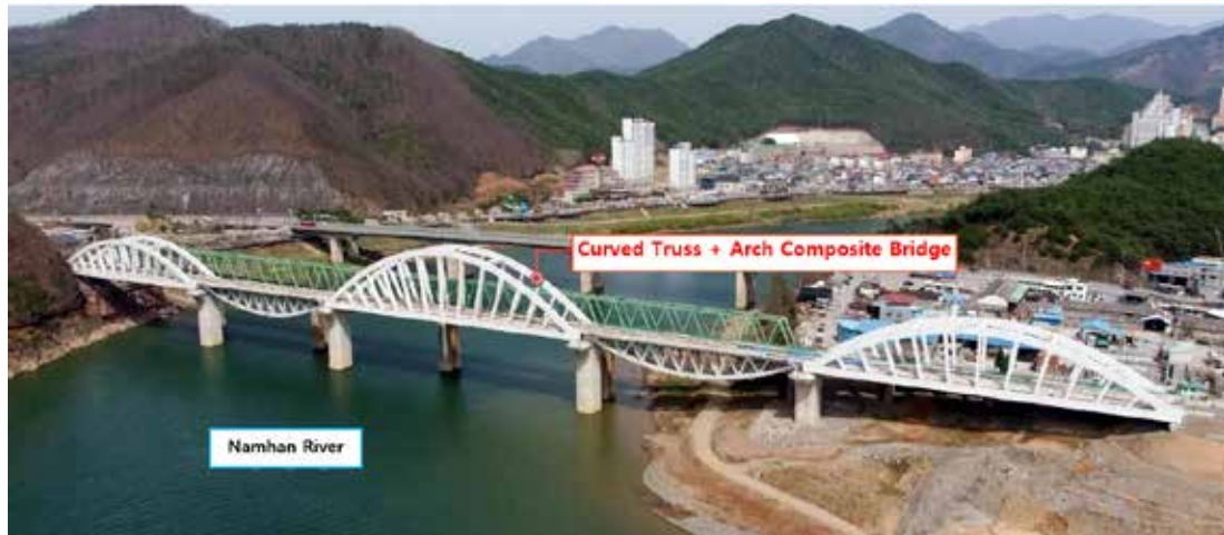
| Figure 2-12 | Panoramic view of the Namhangang Bridge on the Dodam-Yeongcheon double-track railway
